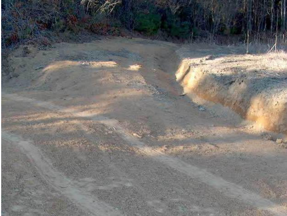
FIGURE 3.3 Typical Turnout
